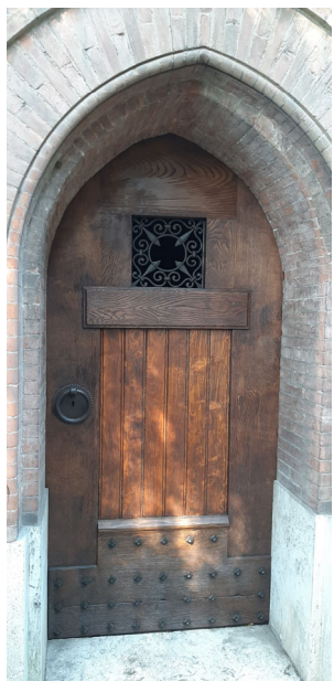
The tower door restored
